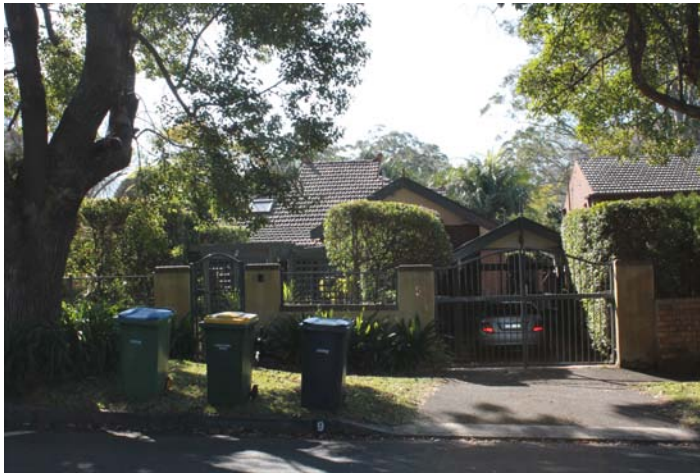
Figure 3.25 Eastern Road Turramurra 9 Brentwood Avenue
