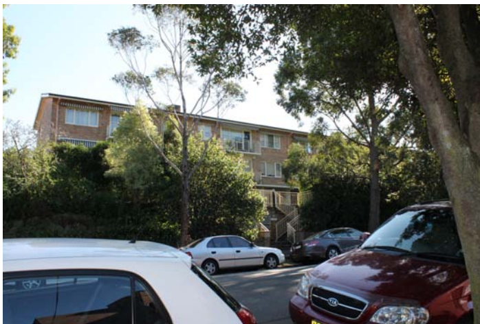
Figure 3.17 Eastern Road Turramurra 26-28 Eastern Road
