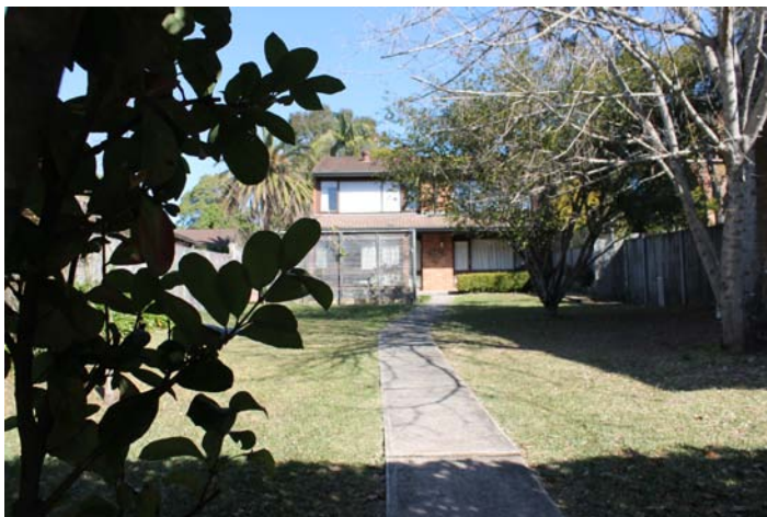
Figure 3.23 Eastern Road Turramurra 6 St. James Lane
