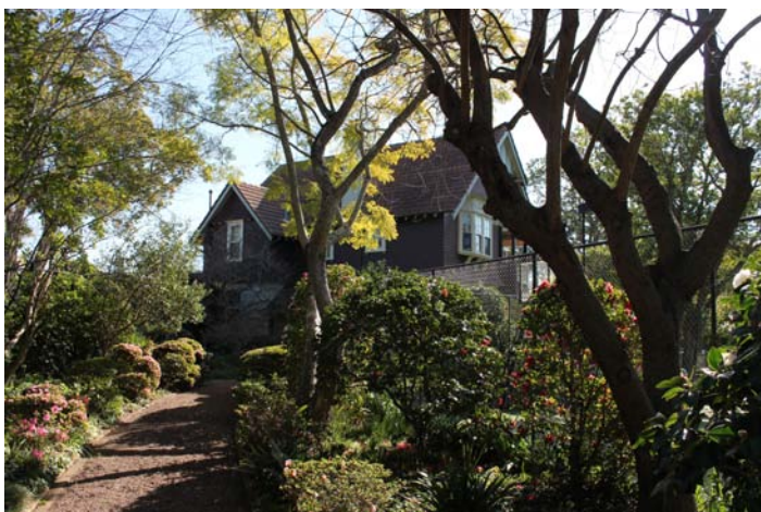
Figure 3.24 Eastern Road Turramurra 46 Eastern Road – signalling the Federation development to the west side of the street
