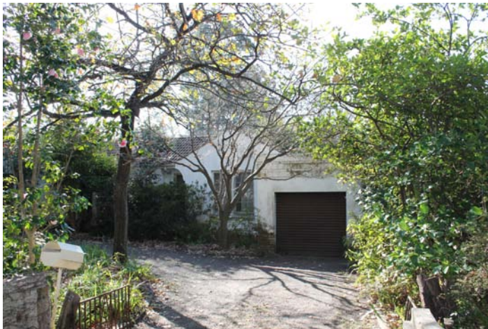
Figure 3.26 Eastern Road Turramurra 5 Brentwood Avenue
